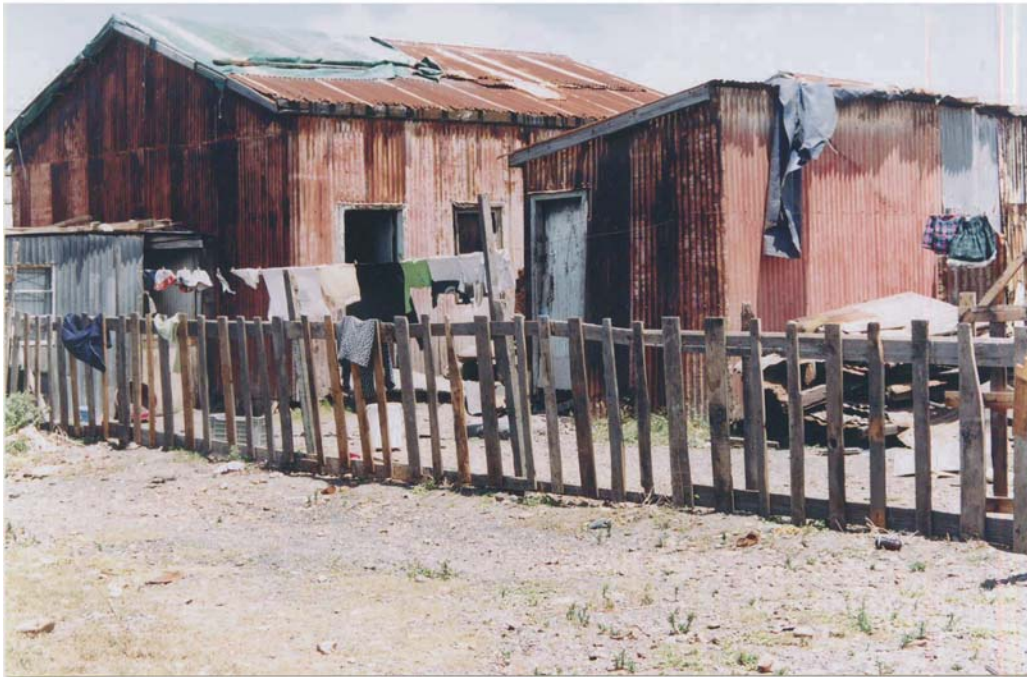
Fig. 2. Houses at the Red Location
